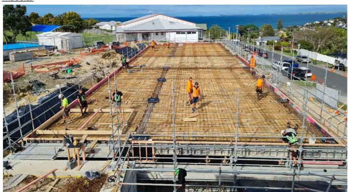
Our New Building has been progressing under Level 3. The Team were able to lay mesh for the first floor over the week and tomorrow will be the day for the concrete pour. You can see updates of the build on the <u>Live Camera</u>.
